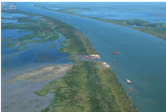
PHOTO: US ARMY CORPS OF ENGINEERS
